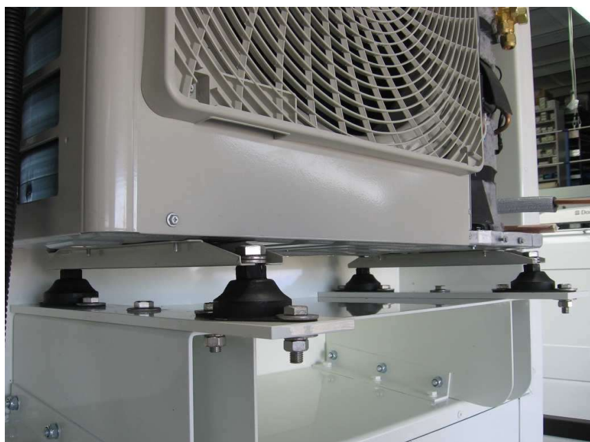
Figure 3: Perfection down to the most minute. All compressors are fitted with the appropriate vibration damper, so that the resulting noise is optimally kept away from the interior
